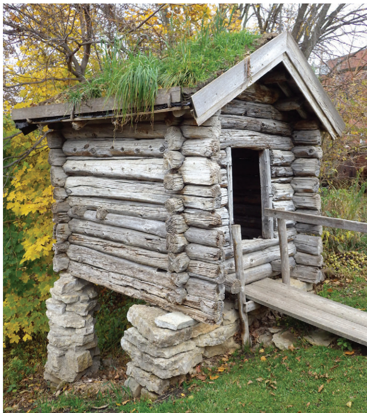
Fig. 3: Norsvin Mill (LC5990) at the Vesterheim Norwegian-American Museum, Decorah, Iowa. Mill has a groundplan of 2.6 m (8 ft, 5 in) by 2.3 m (7 ft, 7 in).
